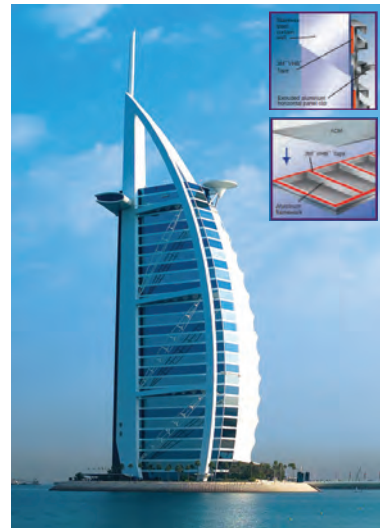
Burj Al Arab Hotel, Dubai UAE Aluminum composite panels bonded to framework to resist high wind loads.
