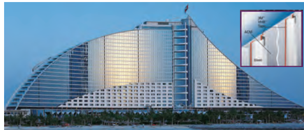
Jumeirah Beach Hotel, Dubai UAE Curtain wall design: Aluminum panels bonded to steel stiffeners.
