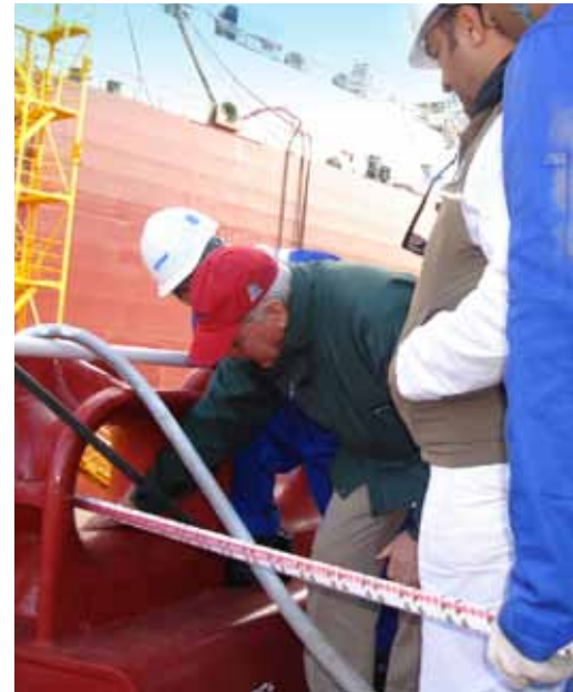
As an integral part of The Samson Advantage, Samson's field technicians provide onboard inspections, repairs, and splicing assistance.
