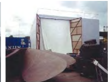
PLYWOOD WAREHOUSE 28 x 15 x 6/6.5 MTR WITH 5 MTR x 6.2 MTR OPENING/DOOR
